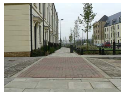
Raised tables and changing textures for pedestrian crossings
