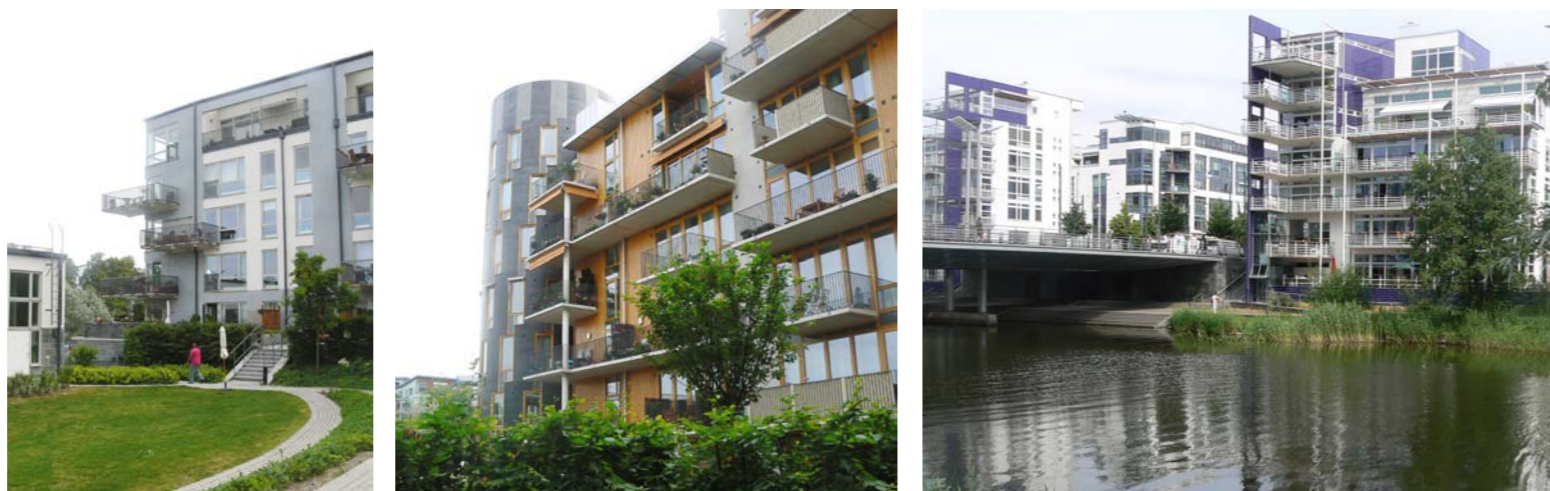
These images of Hammarby, Sweden show the variety of building forms within a single development
