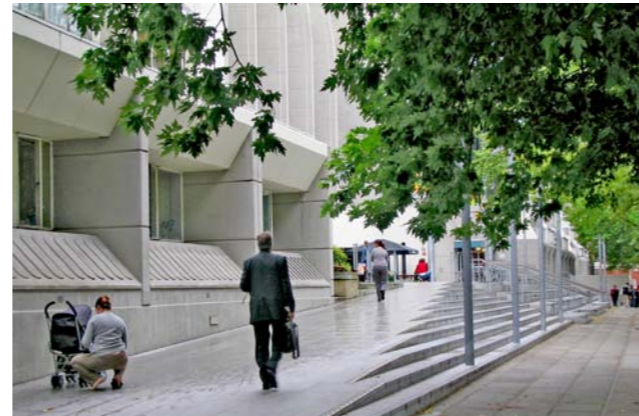
Integration of stairs and ramps at the Brunswick Centre, London
