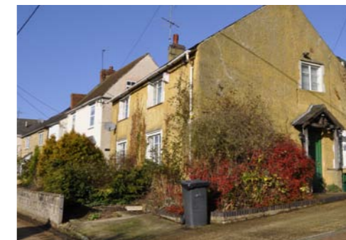
A similar house layout in Greens Norton with access to the building from a side entrance whilst the main frontage faces the street
