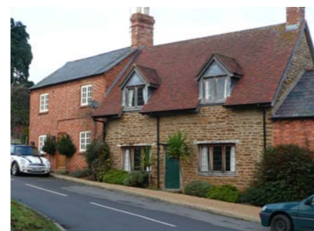
Architectural features and use of local materials add to the townscape quality and character of a village
