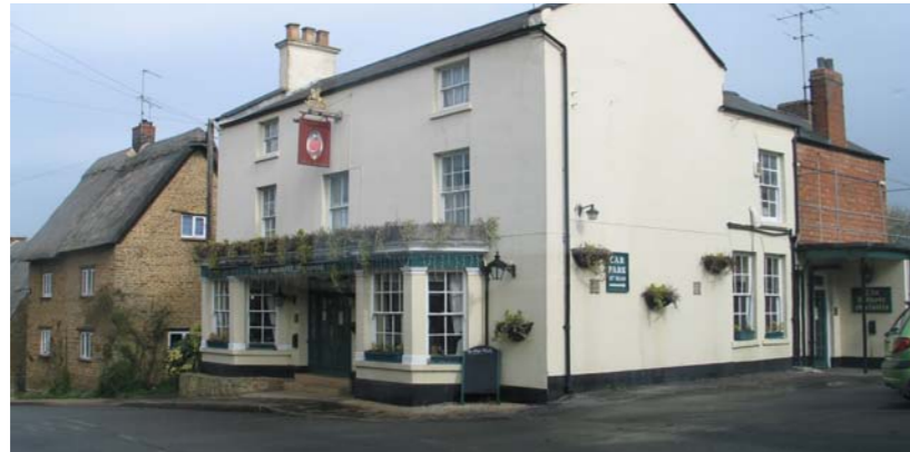
Village centres often contain a public house, one of the few surviving village amenities
