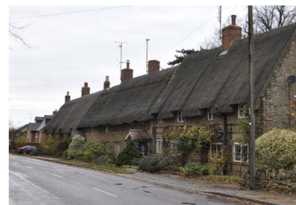
Defined line of thatched roofed houses provide definition to the street
