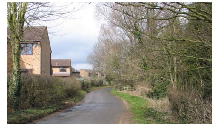
Buildings back off from the rural edge with hedges and a lane demarcating the boundary of the built areas
