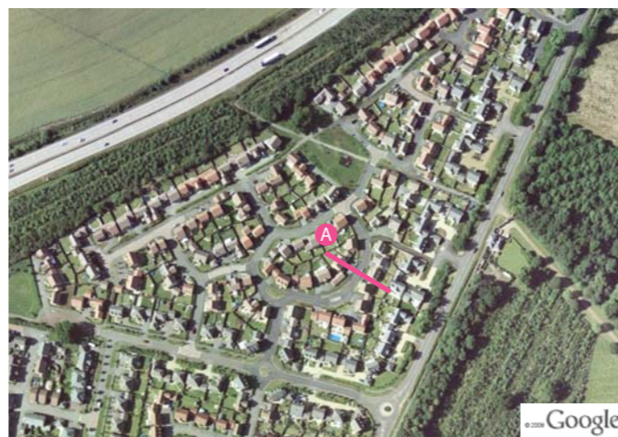
Figure 164 : Aerial image of a suburban recent development
