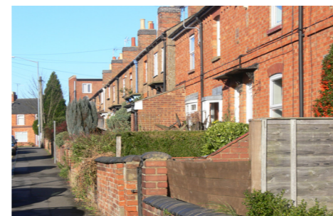
Streetscape defined by consistent massing and texture on building frontage.
