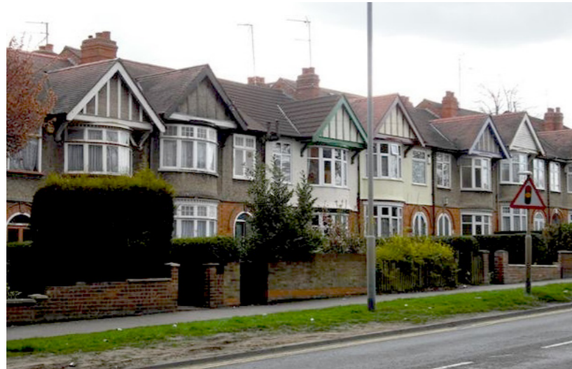
Buildings aligned on slope
