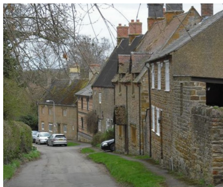
Dramatic streetscape in Newnham as a result of a street that cuts across the contour
