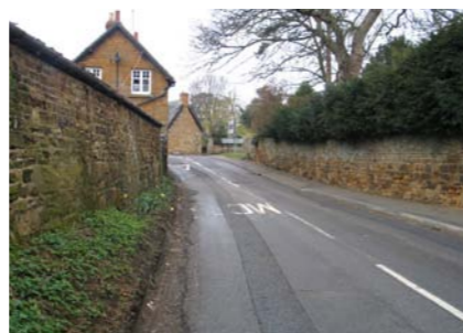
Main movement route enclosed by boundary walls and landscaping
