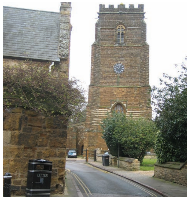
Historical buildings such as the Town Church in Towcester, were constructed in the locally sourced ironstone
