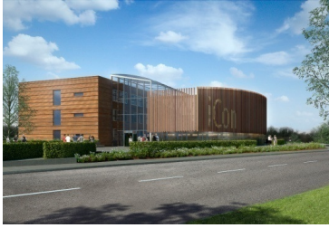
The iCon, under construction in Daventry
