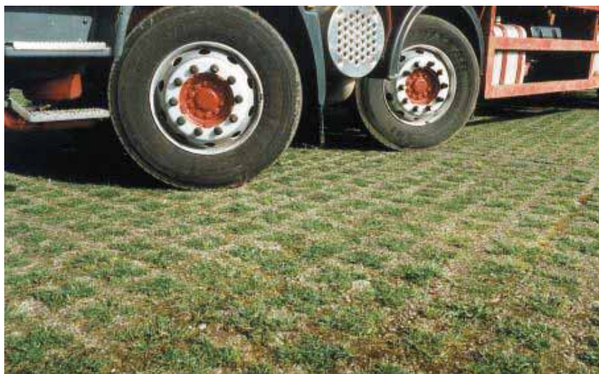
Photograph of a Grasscrete System of permeable paving.
