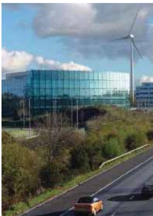
Greenpark 2MWe wind turbine – Ecotricity
