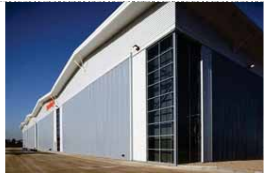
Photograph of the Solar wall system integrated in the Sainsbury's Distribution Centre at Pineham.
