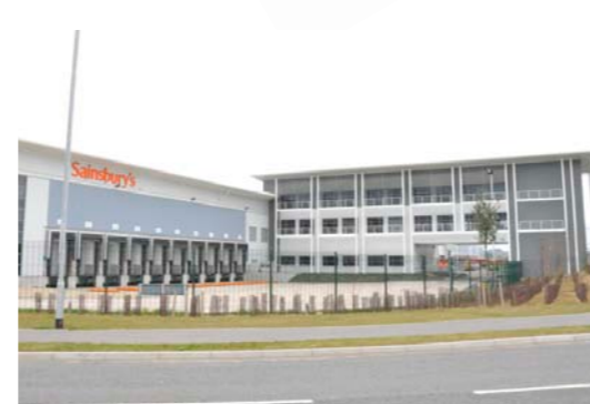
Location of the office unit to the front creating a sense of arrival to the site
