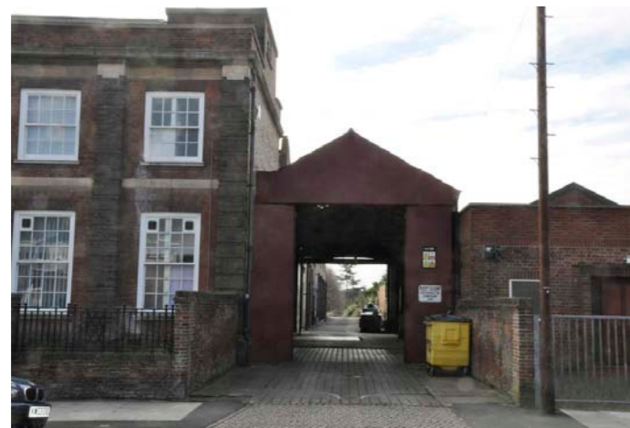
Entrance to parking and loading area from Christ Church Road
