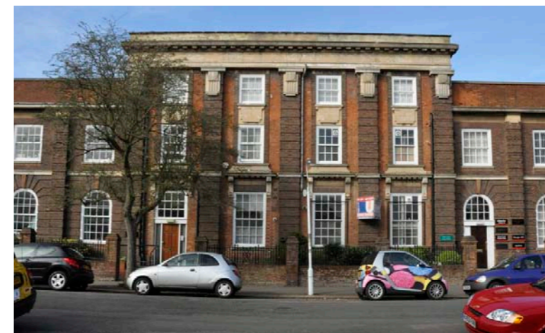
Elevation on Ardington Road, with an enhanced frontage highlighting secondary entrances and frequent fenestration
