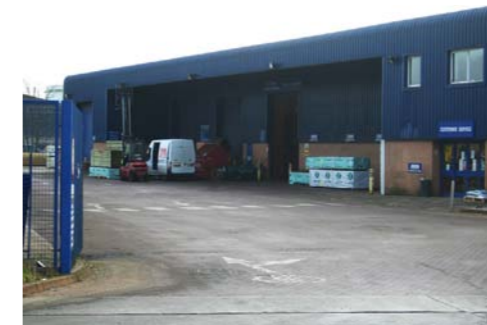
Servicing functions and entrance adjoining each other
