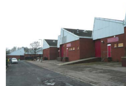
Aligned buildings with no active frontage in Daventry
