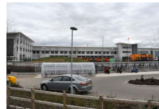
Parking area in proximity of the office unit and including a store for bicycles and motorbikes
