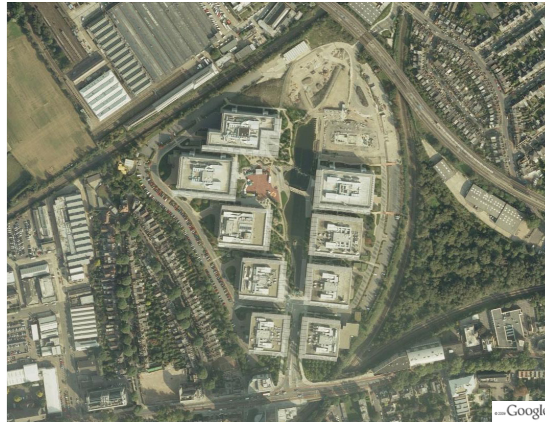
Figure 251: Aerial view showing dense site layout and relationship to adjacent areas and public transport connections (site under construction)
