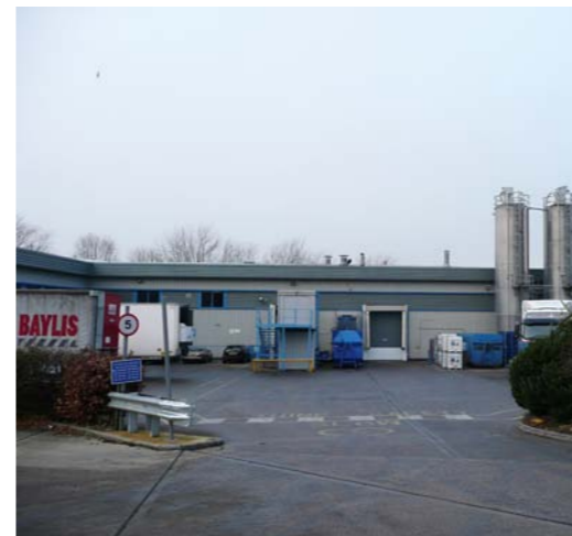
Manufacture and servicing premises in Daventry
