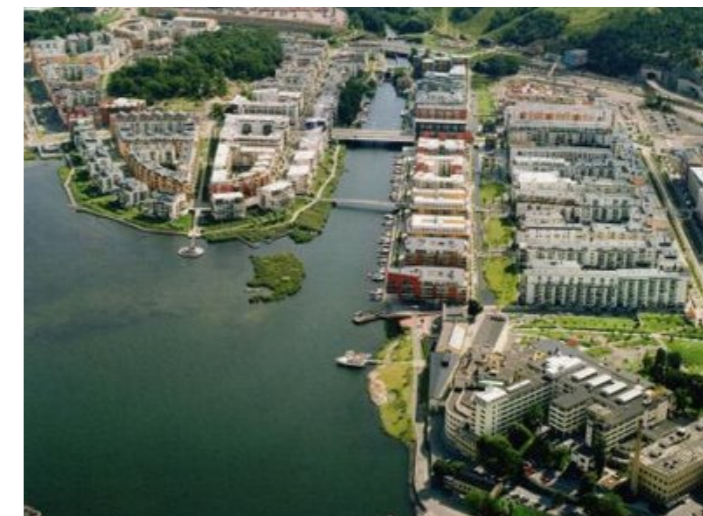
The canal network forms an intrinsic part of the master plan. Source: CABE
