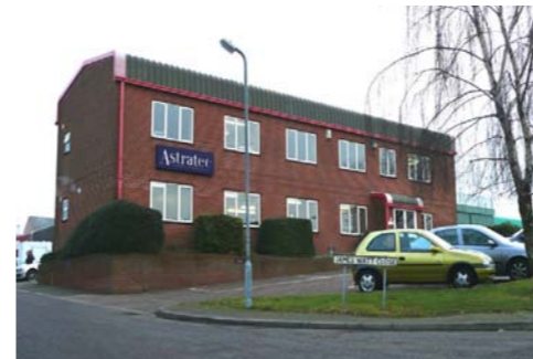
Office building in Drayton Fields employment area, to the north of Daventry
