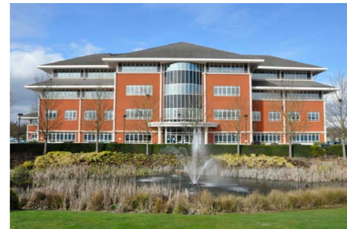
One of the main office blocks characterised by generous fenestration and formal landscape area which creates a setting and sense of arrival to the building.
