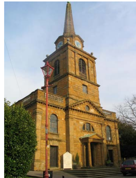
Landmark buildings and markers contribute to overall townscape and improve legibility
