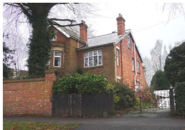
Detached house set back from the street
