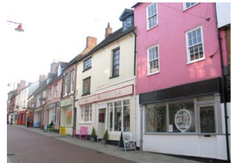
Continuity in roof line and building line unifies the overall street despite variation in individual frontages
