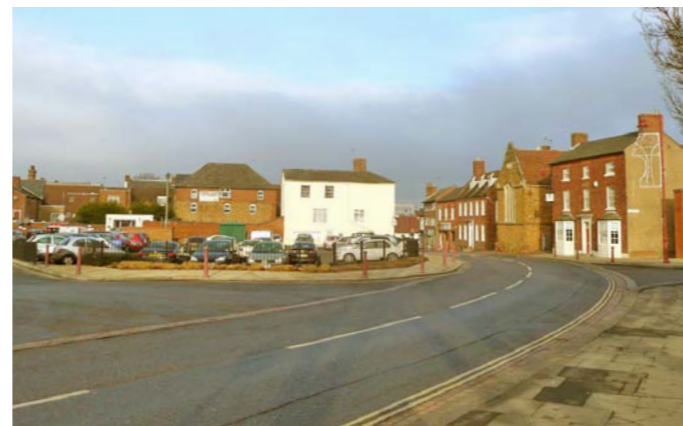
Transition zones can lack character as undefined spaces which are at times used for parking as in this case
