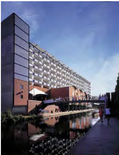
Multi-storey car park, Brindley Place
